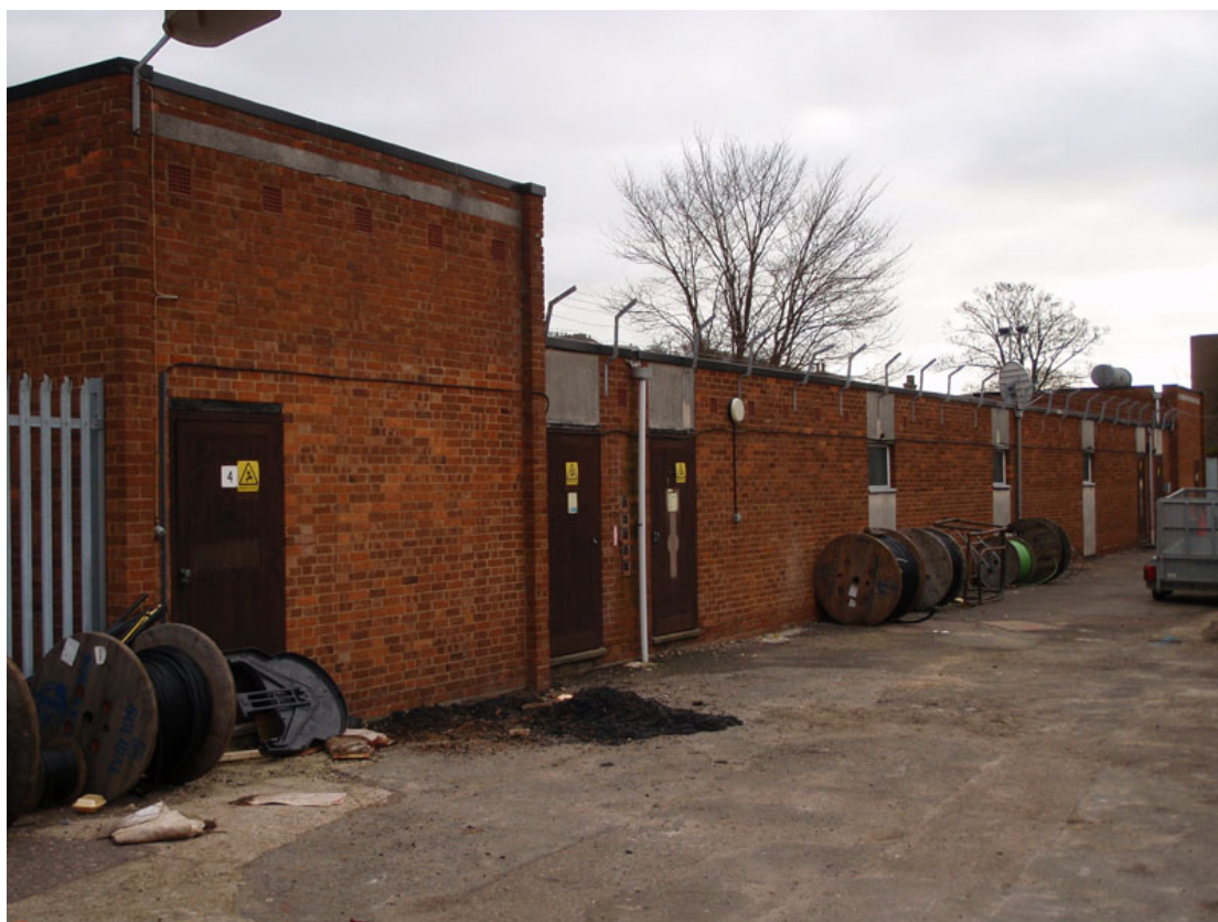
Plate 2. Main Substation Building (looking South East).
