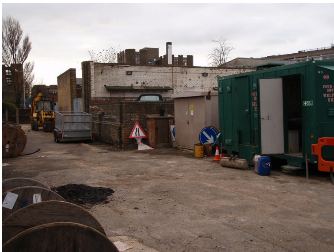
Plate 3. Part of Substation Compound (looking South).
